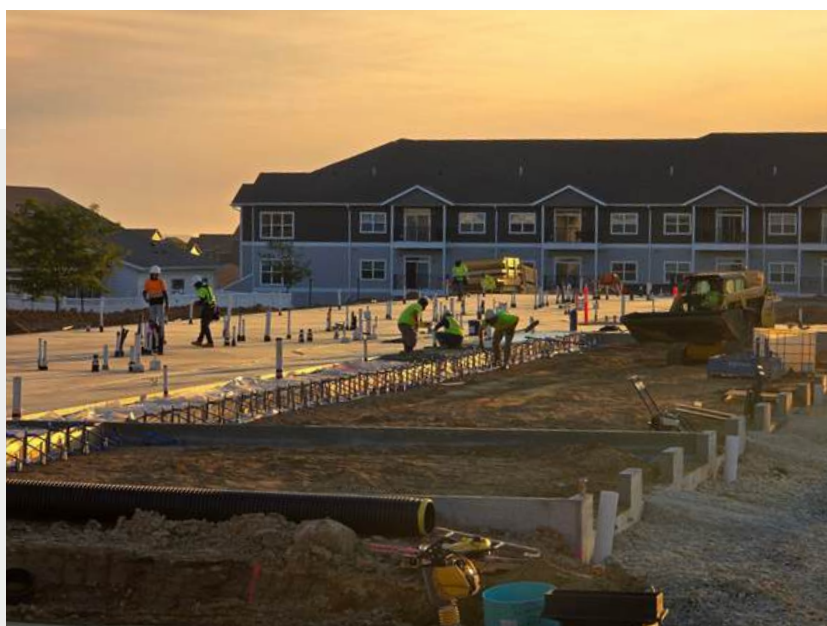
Construction progress from October 3, 2024
