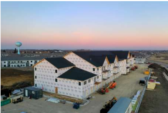
Stone Haven Apartments construction progress.
