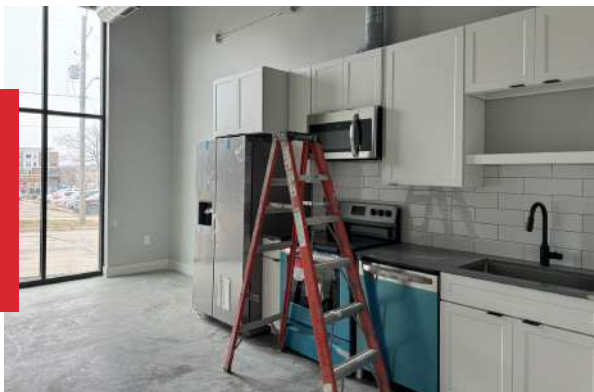
Construction of an industrial flat in March
